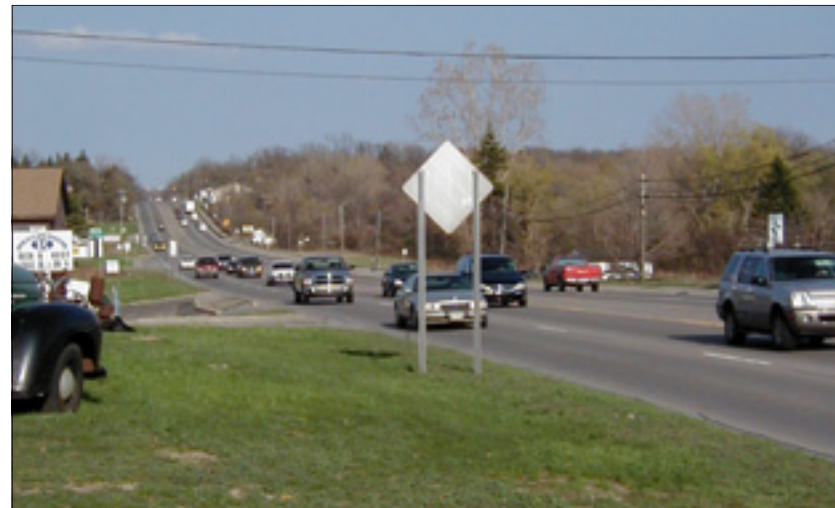
Highland Road, looking east. Integrating and coordinating pathway, pedestrian amenities, landscaping, boulevards and entry signs are techniques that will announce to visitors that they have entered the White Lake Township community.
