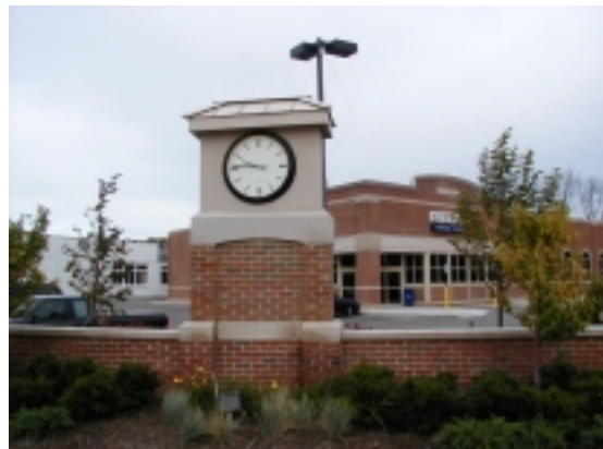
Amenities such as decorative walls and landscaping serve to partially screen parking areas and provide an attractive front yard and side yard area.
