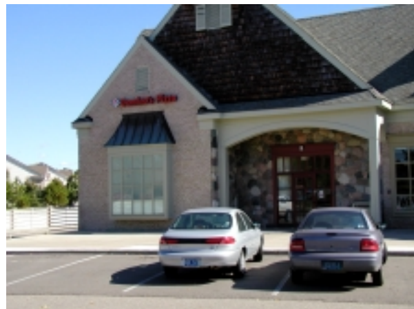
This Domino's Pizza has an understated appearance, producing a unified look with the main center.
